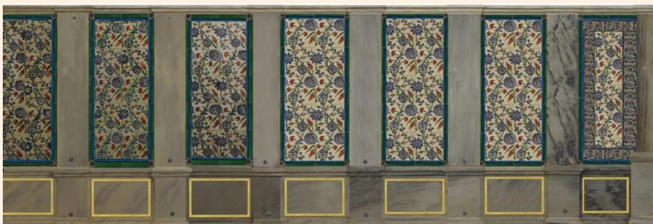
Part of Qibla wall after restoration
