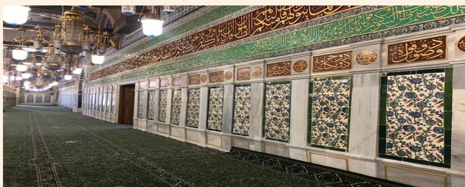
Qibla wall after restoration
