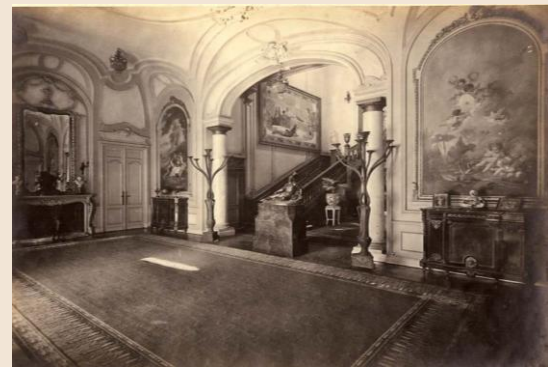
Main entrance Hall
