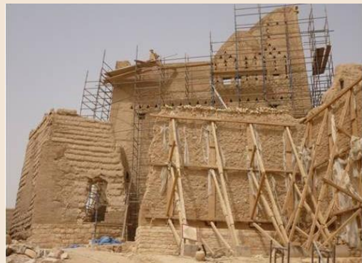
Salwa Palace Shoring works
