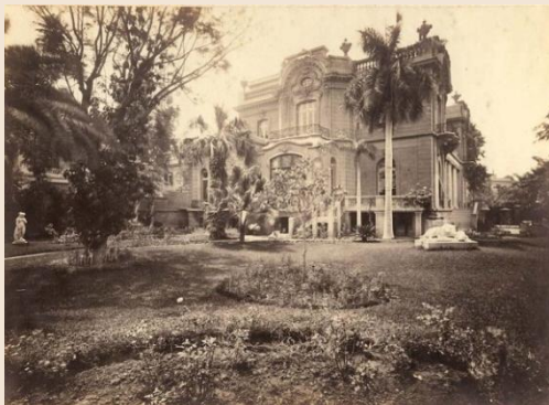
North façade and garden
