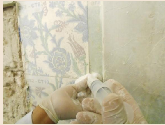
Consolidation of mortar with Ledan
