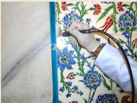
Cleaning of ceramic tiles
