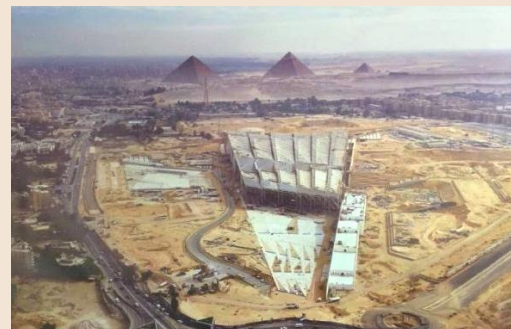
Museum during construction
