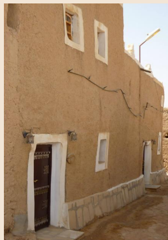
Restored house at Al-Ḥala village
