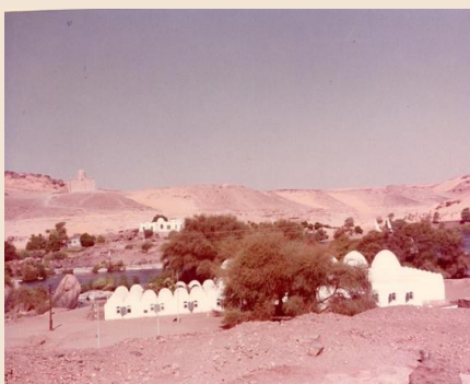
Site General view
