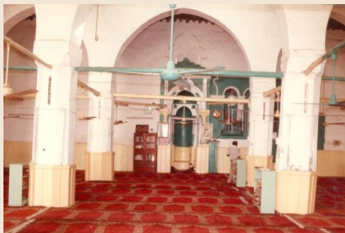
Qibla wall-dampness in columns- CIAH 1985
