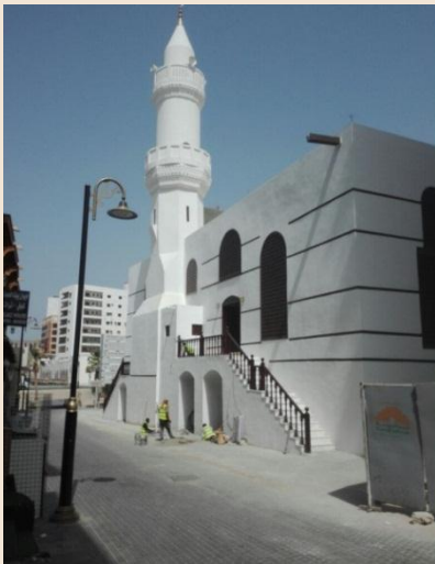
South façade after restoration
