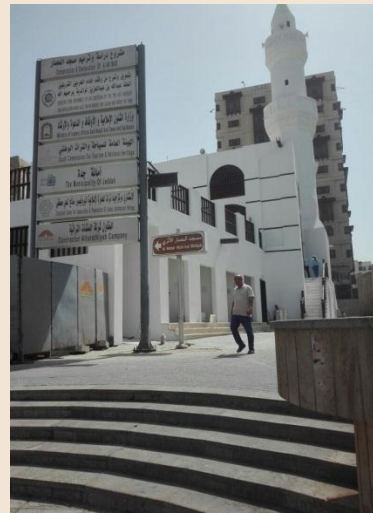
South façade after restoration
