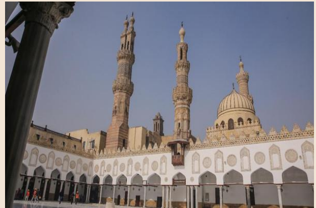
Sahn after restoration
