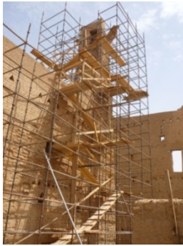
Salwa Palace - tower during restoration
