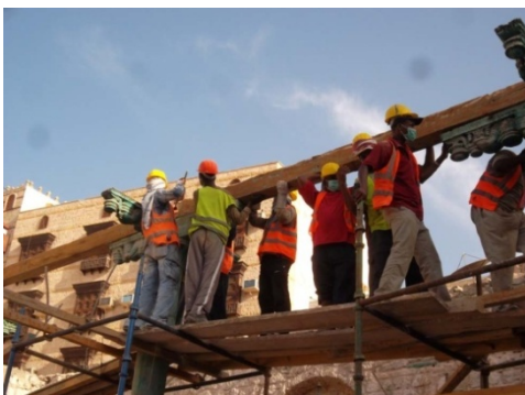
Laying girders of Riwāq
