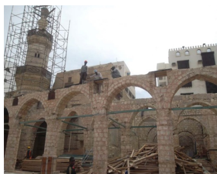
South Riwāqs during restoration
