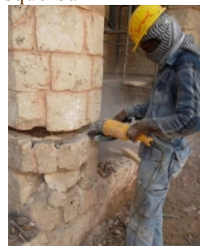
Removing deteriorated wooden rings
