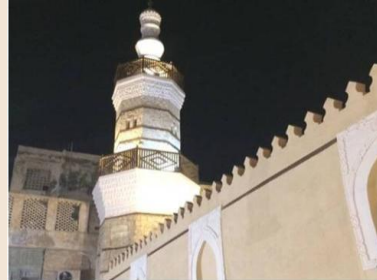
Minaret after restoration
