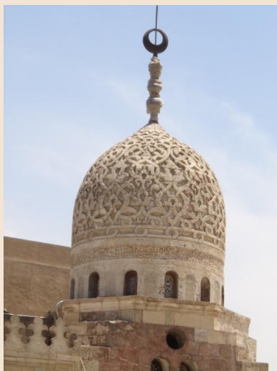
Dome after restoration Gawhariyya madrasa
