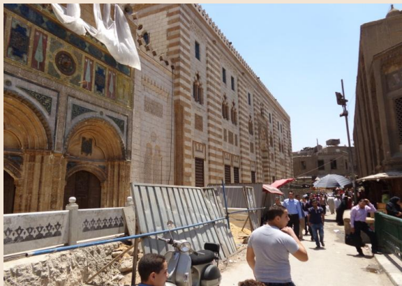
North West Elevation-during restoration
