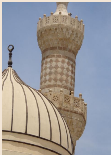
Dome and minaret after restoration Aqbaghawiyya Madrasa
