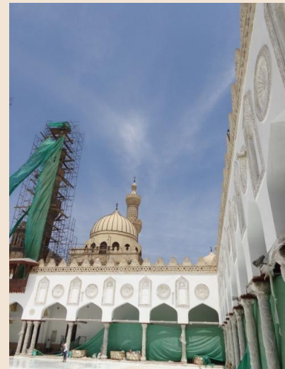
Sahn during restoration
