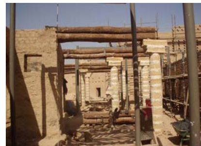
Omar Palace - Installing main wooden girders
