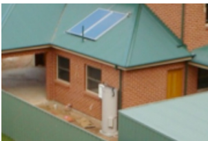
Split system solar
