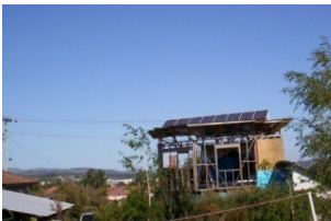
Flat roof on frames
