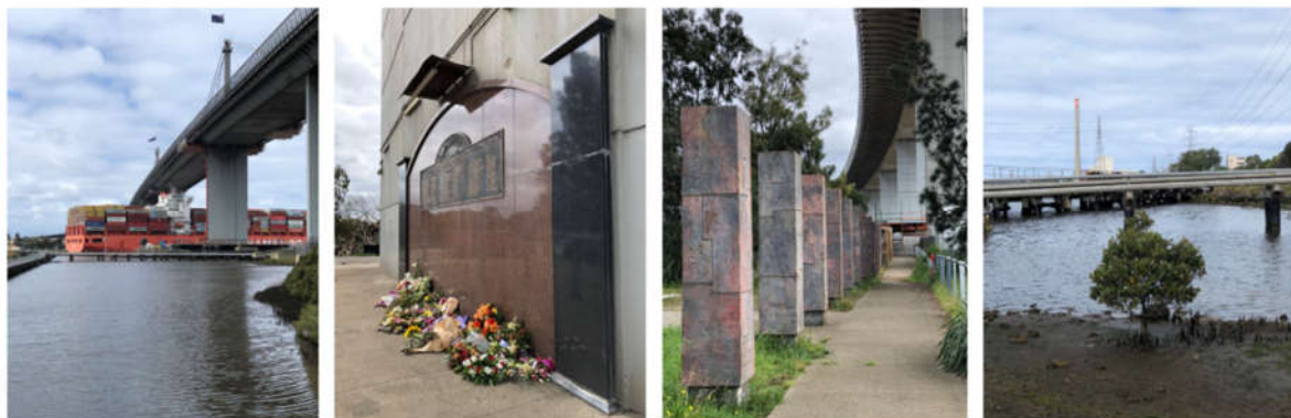
Westgate Bridge and Stony Creek Backwash
