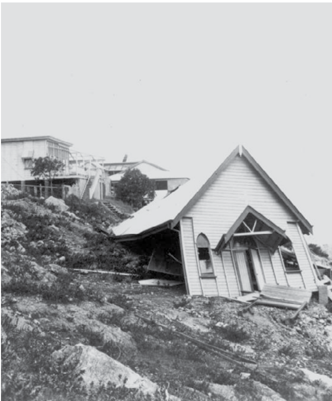
Destruction of Chinese Mission Hall in Townsville caused by cyclone Leonta, 1903: John Oxley Library, State Library of Queensland, D10-10-89
