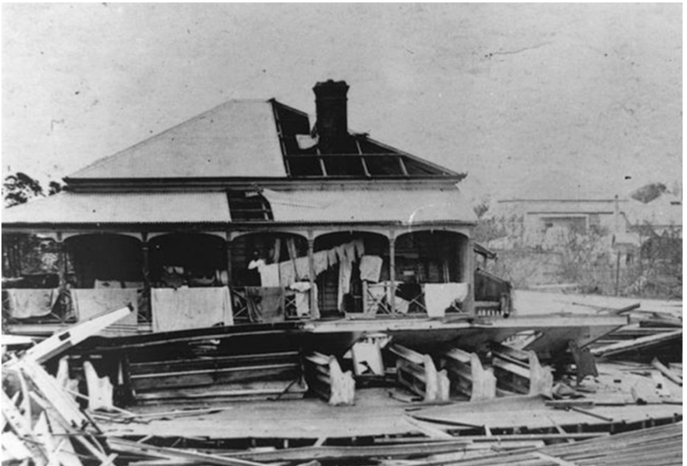
Cyclone damaged Methodist Church at Mackay (Queensland, Australia) 1918. This image depicts the flattened Methodist Church on Gregory Street, Mackay and the damaged Parsonage next door. (Image: John Oxley Library, State Library of Queensland)
