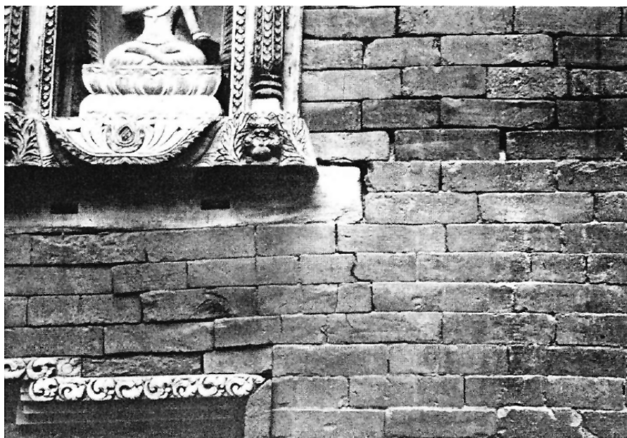
Fig. 8. Variations in brick joints between a niche and a door sill as a result of different compressive forces. This sill has also had timber replaced with brick tile.
