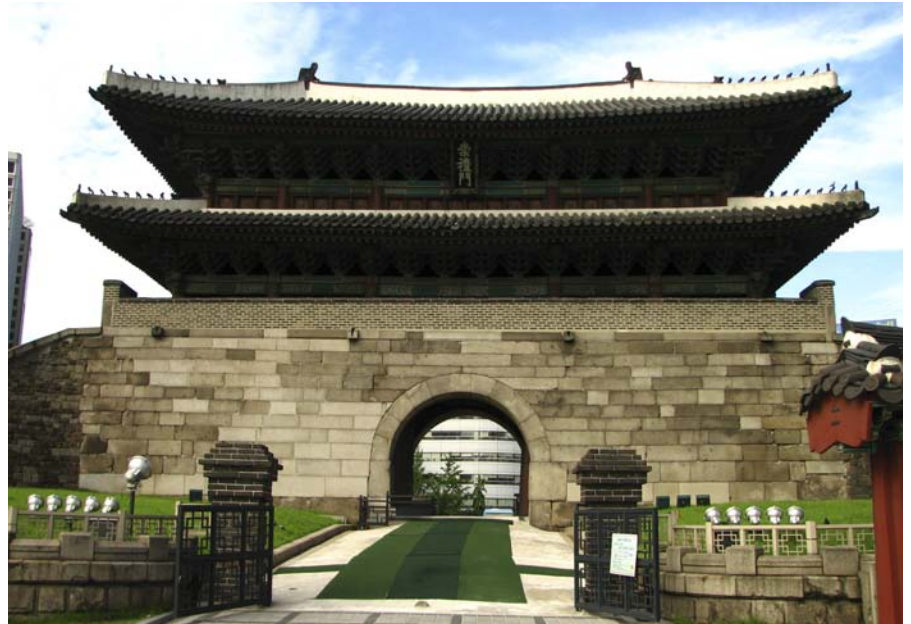
Sungnyemun Gate before the 2008 fire.
