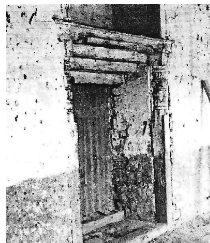
Fig. 5. Rear view of an upper floor window opening. The floor joists and wall plate are visible at the top.
