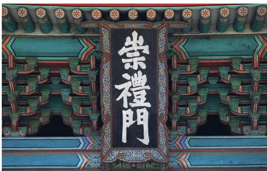
The signboard of the gate, after restoration.
