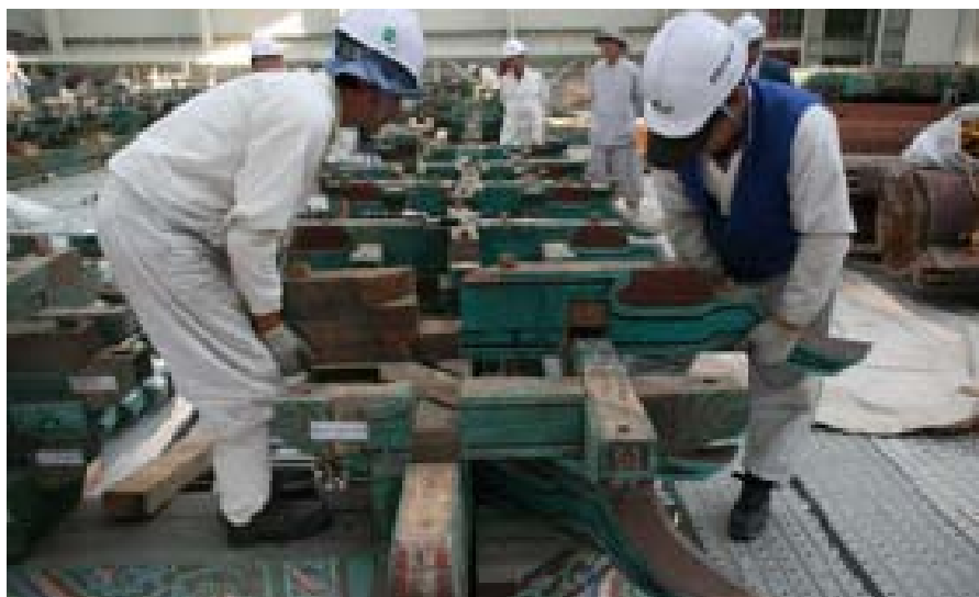
Reassembling the wooden pavilion-lower floor (photo: Shin, Eung-Su).
