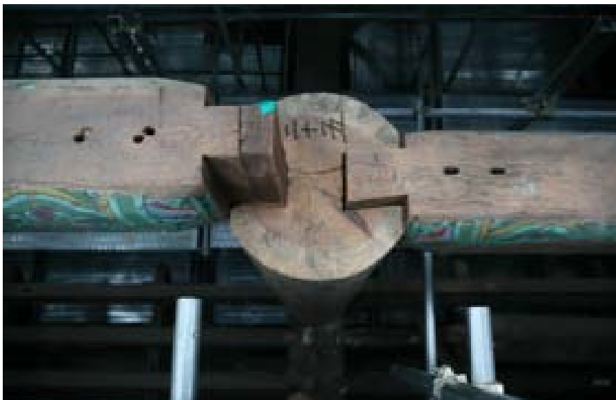
Both the salvaged (connection beam) and new (column) wood were used (photo: Shin, Eung-Su).
