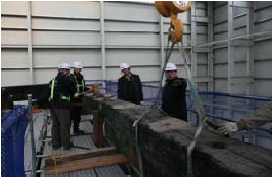
Disassembling the salvaged parts, 2009 (photo: Shin, Eung-Su).
