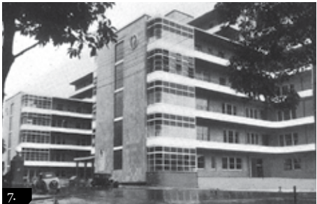
1941 King George V Memorial Hospital, Camperdown Architect: Stephenson, Meldrum and Turner Award: Sulman Medal, 1941. Listed: Sydney LEP
