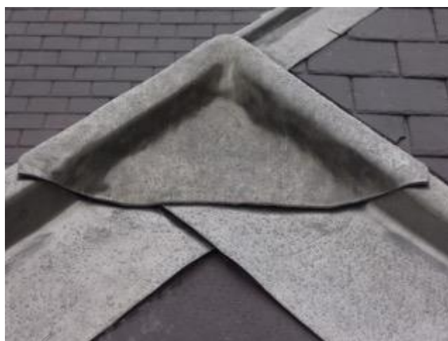
Lead cappings on slate roof – Fire Station, NSW
